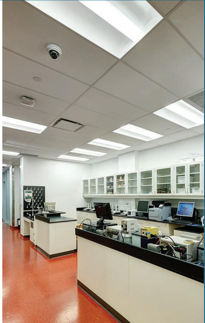
In ESCB's laboratories, ROCKFON Medical Plus ceiling panels meet stringent requirements for clean room environments and contamination control, as well as repel harmful microorganisms, mold and bacteria. These ceiling panels also withstand high humidity and rigorous cleaning.
