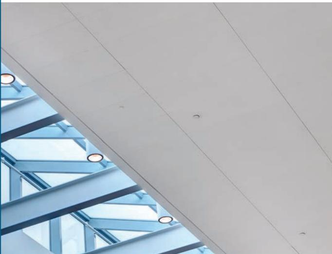
Throughout the atrium, corridors and faculty offices, ROCKFON Artic ceiling panels feature shiplap edge details and custom sizes, installed with hairline precision to give the appearance of a smooth, continuous ceiling.
