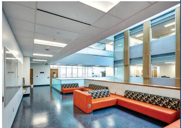
Throughout ESCB's corridors, ROCKFON Artic ceiling panels were installed in Chicago Metallic 1200 Series exposed 15/16-inch ceiling suspension system. When maintenance is needed, it is easy to remove one or several ceiling panels to gain access to the plenum and to return them without damage.
